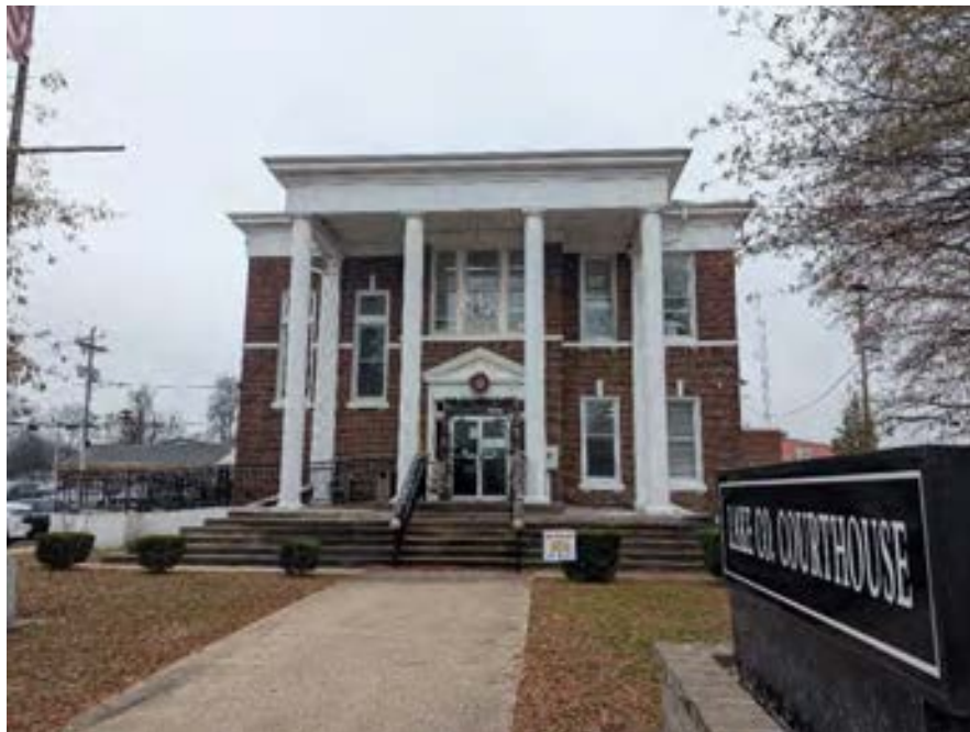
Figure 2: Lake County Courthouse (Front)
