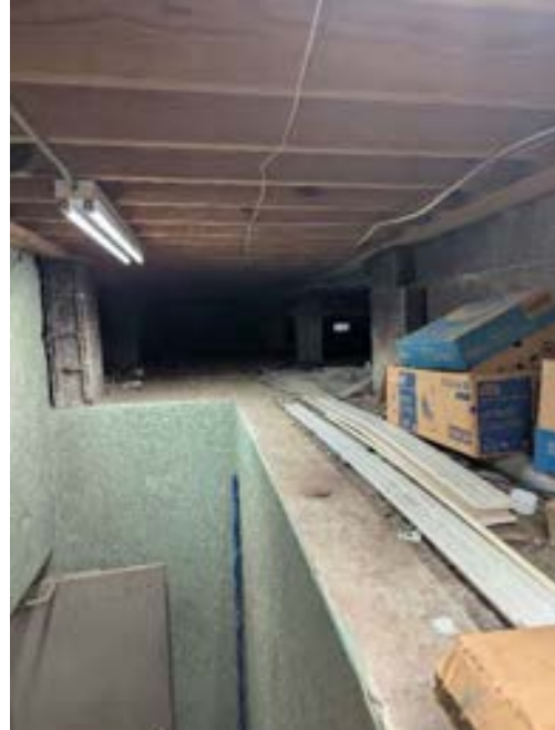
Figure 5: Current Basement Roof Insulation
